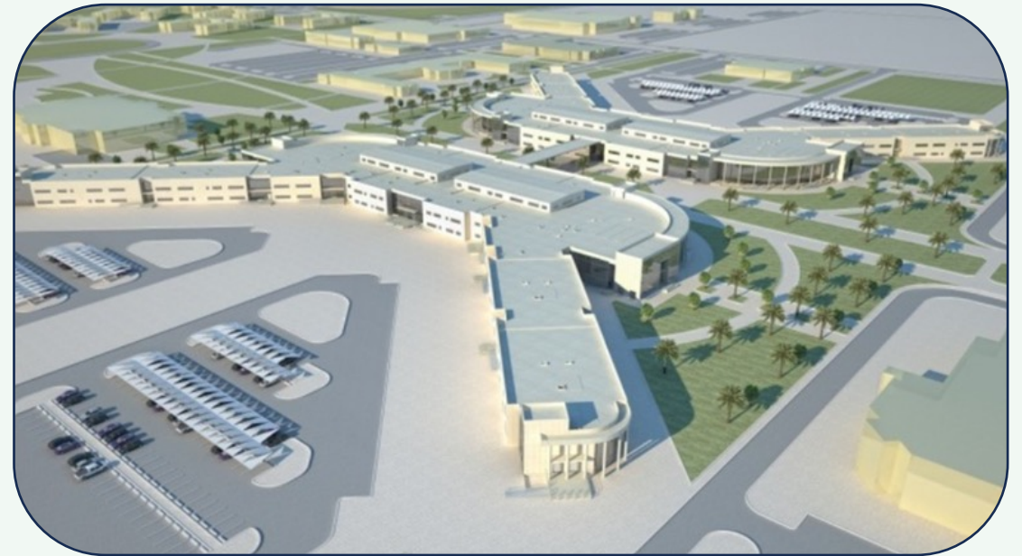
120 Buildings — King Faisal Air Academy
